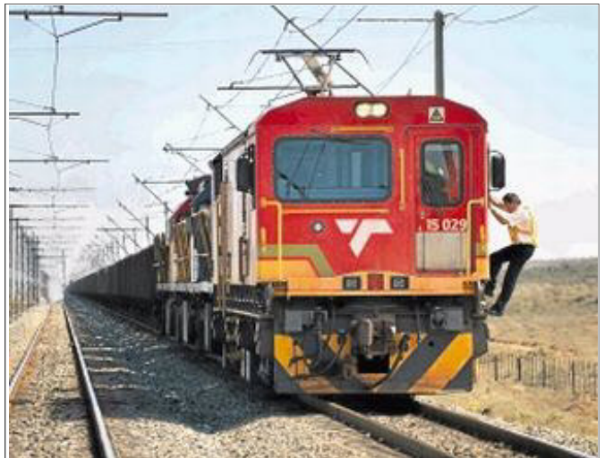
SMOOTH OPERATOR: One of the brand-new Ore Line locomotives at the head of a 40 000-ton ore train north of Saldanha. The new trains boasts air-conditioning and state-of-the-art computers
